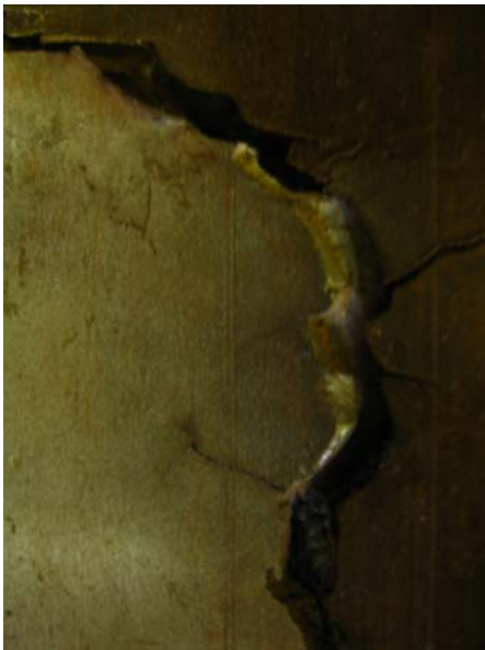
Figure 3: Example of sulfide stress cracking
